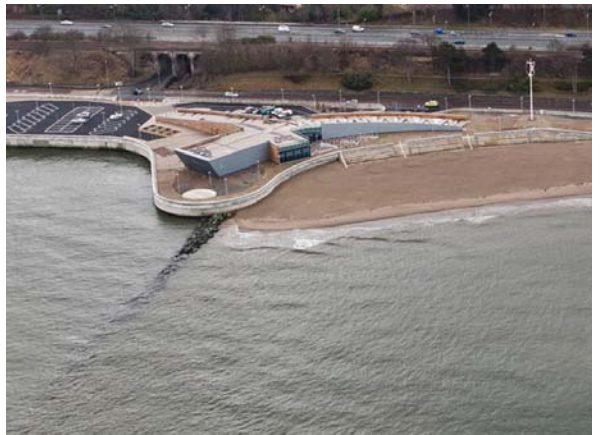
The new Porth Eirias building was built by Wynne Construction
